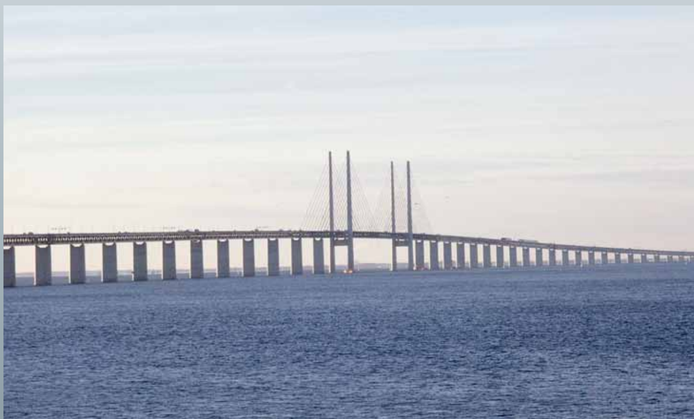
The Öresund Bridge
